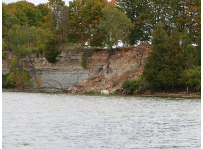
Figure 18: Bedrock Cliff Collapse where the Bill's Creek Shale has undercut the Overhanging Stonington Limestone North of Stop 3. Photo by Dave Adler.
