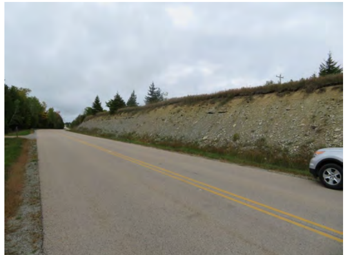
Figure 6: Roadcut Along CO 513 Looking North. Note Gray Bill's Creek Shale Overlain by Tan Stonington Limestone. The Entrance to Lakewood Cemetery is in Middle Left of Photo. Photo by Dave Adler.
